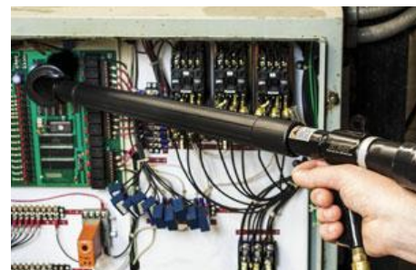
Model 6292 Vac-u-Gun Transfer System carries dust away from sensitive electronic controls.
